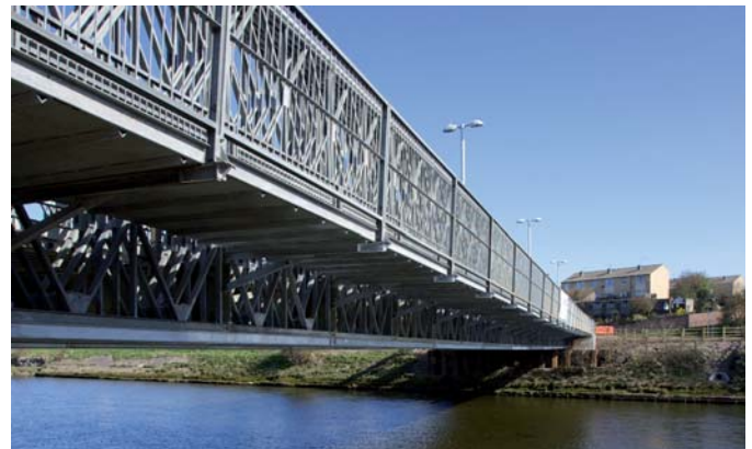
Above: A new two-lane temporary road bridge capable of taking HGVs was opened in Workington on April 21st. It took contractor Morgan Est just 72 days to build.
