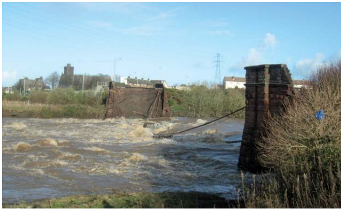
Above: Northside bridge in Workington collapsed at the height of the floods, killing PC Bill Barker and cutting off communities either side of the river.
